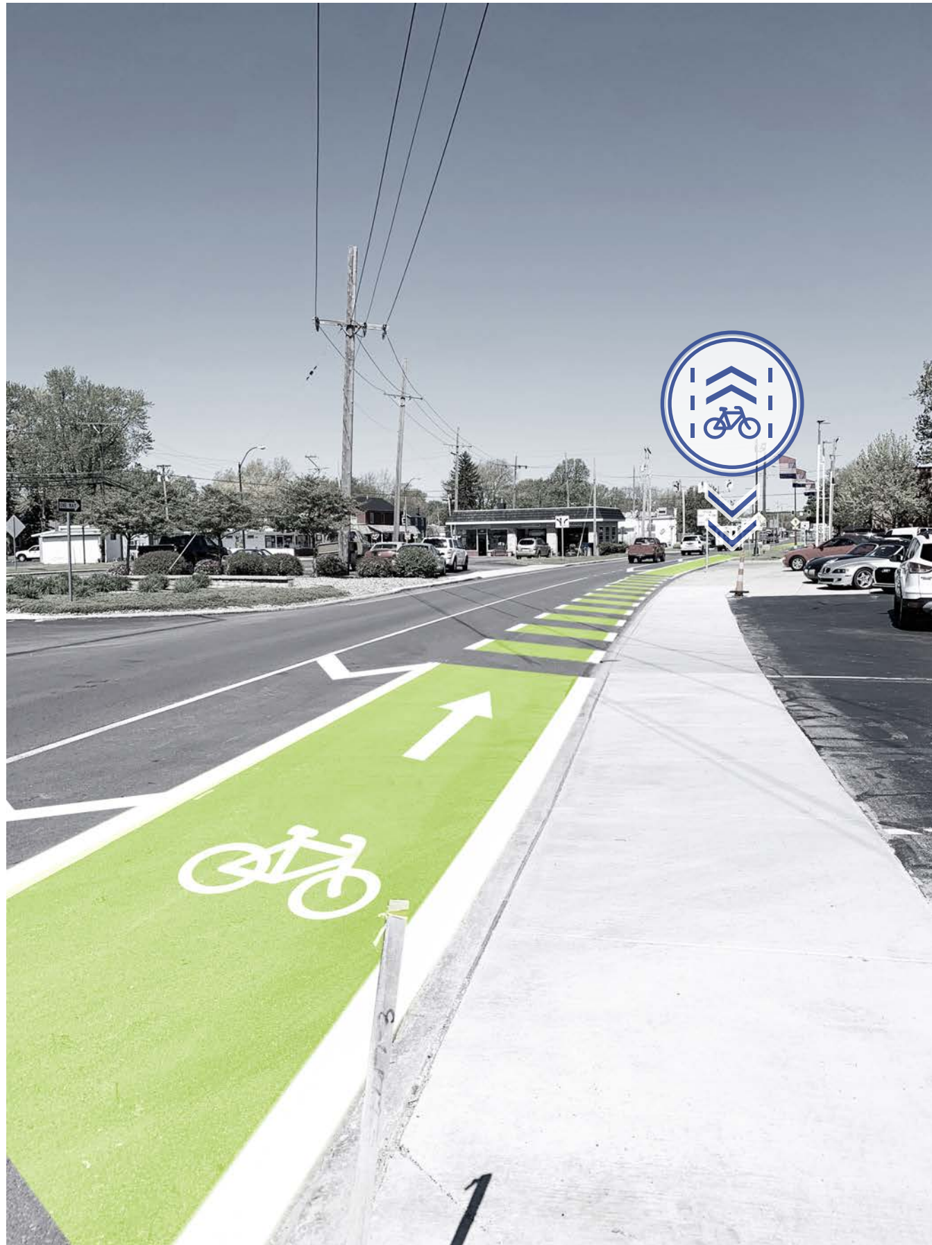
Painted bike lane delineation looking west toward Huron Street. The updated configuration includes a continuous bike lane, shaded and dashed through the Huron St. intersection.
