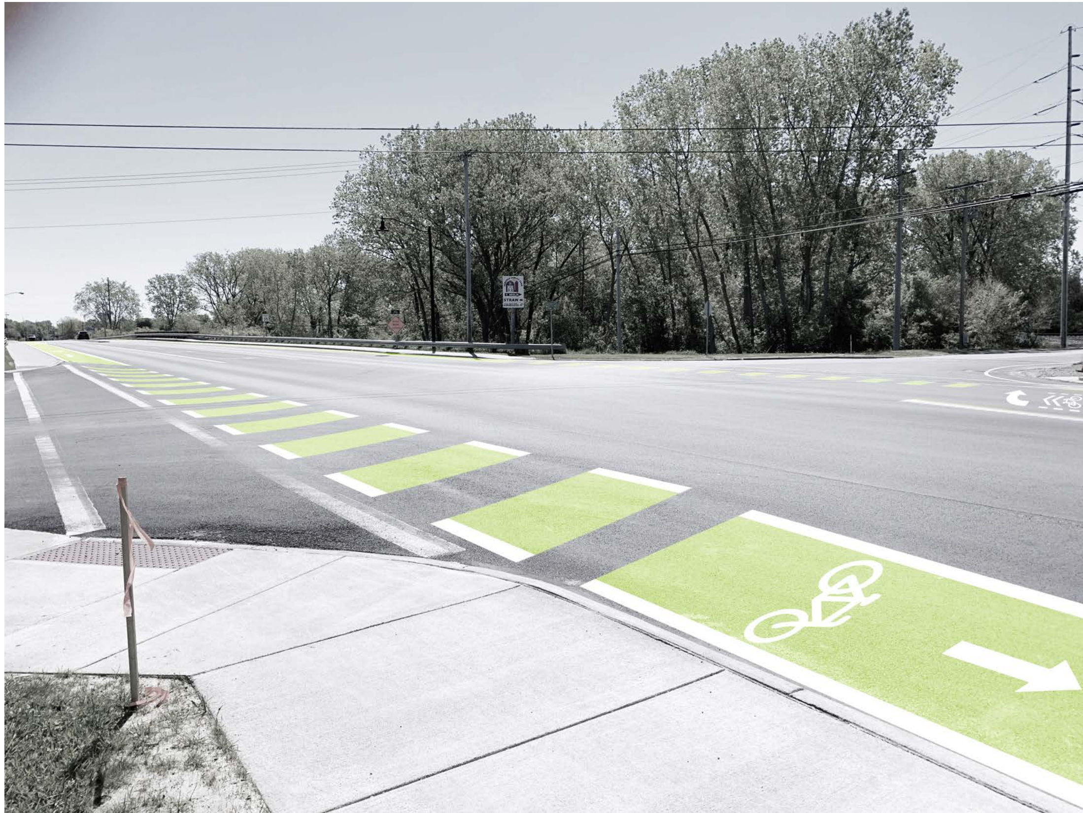
Painted striped bike lane adjacent to crosswalk at the intersection of River Rd and US 6 looking southeast toward Berlin Rd. The updated eastbound lane incorporates a shared turn lane onto River Rd.
