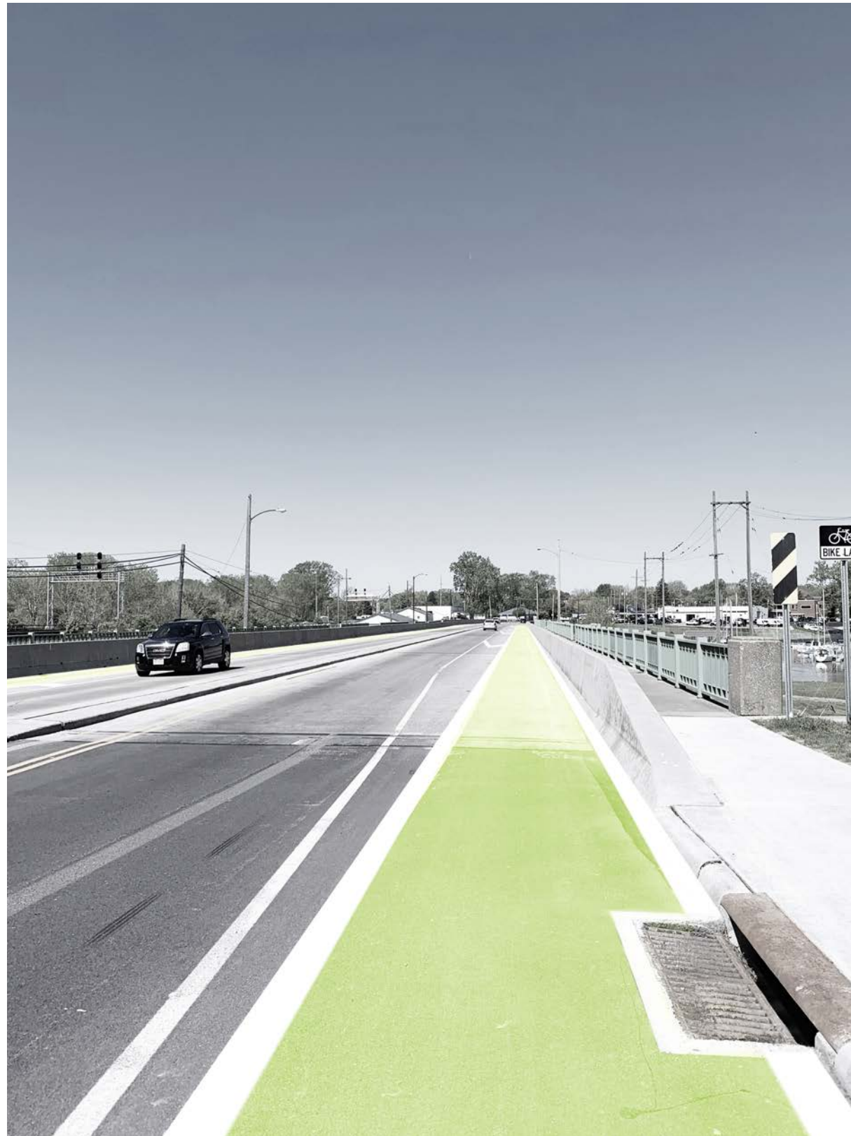
Painted bike lane delineation with striped buffer pproaching the Huron River bridge - view looking west toward Downtown
