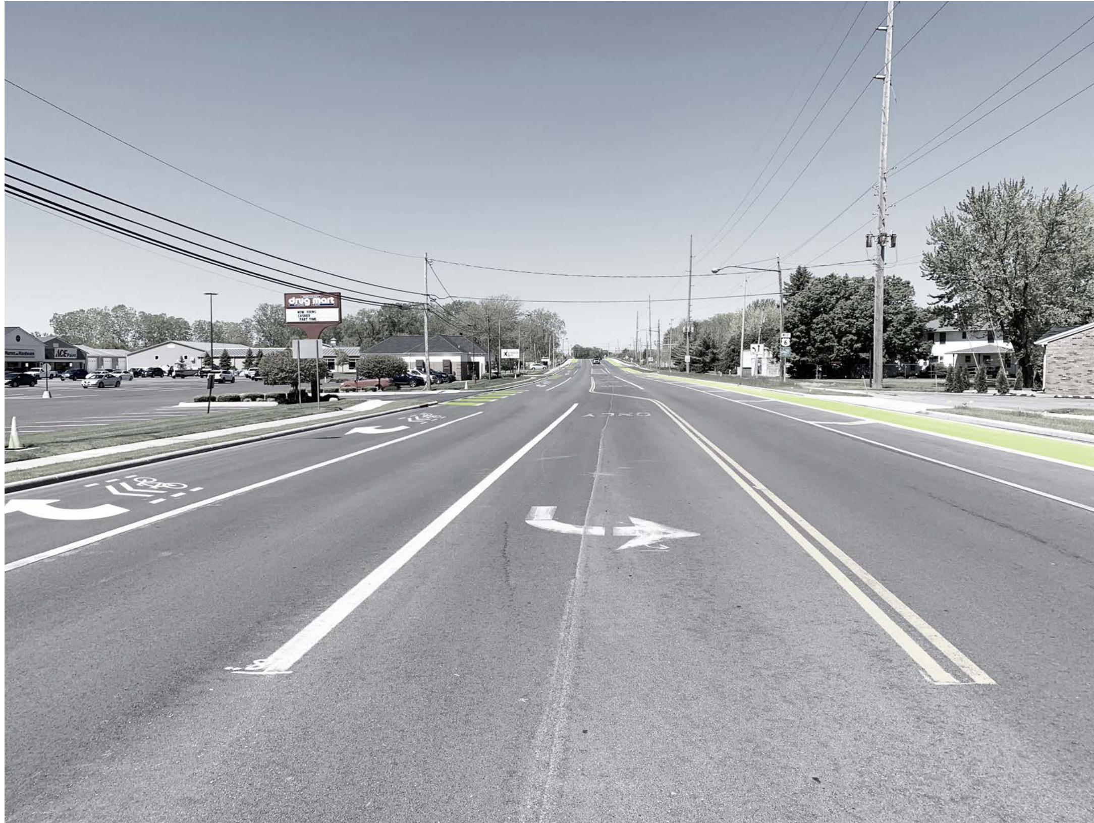
Painted striping and shared turn lanes to indicate delineation of separate protected bike lane from motorist traffic at the intersection of Berlin Rd - view looking west toward Downtown. Eastbound traffic has been updated to include shared turn lanes and bike lane striping at intersections and drive aisle entrances.
