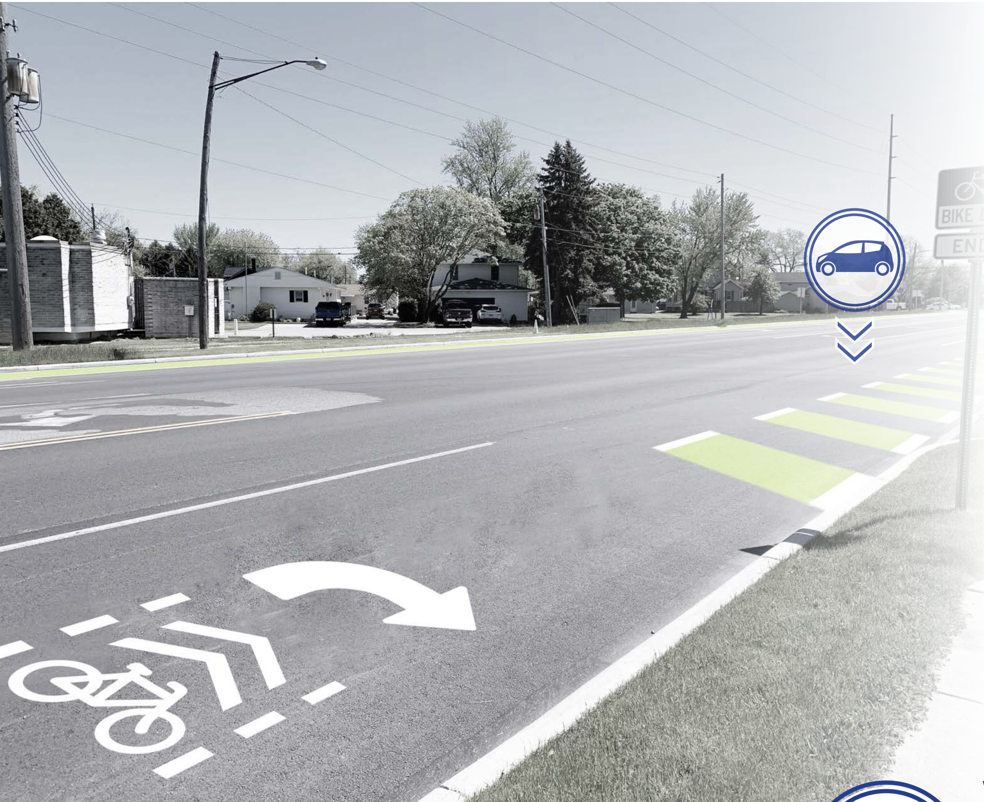
Painted striping to indicate merging of the bike lane back into motorist traffic - looking east at the Commerce Plaza entrance - view looking toward Berlin Rd. The updated configuration features continuous shared turn lanes with dashed bike lane indicator striping through intersections and along curb cut frontages.
