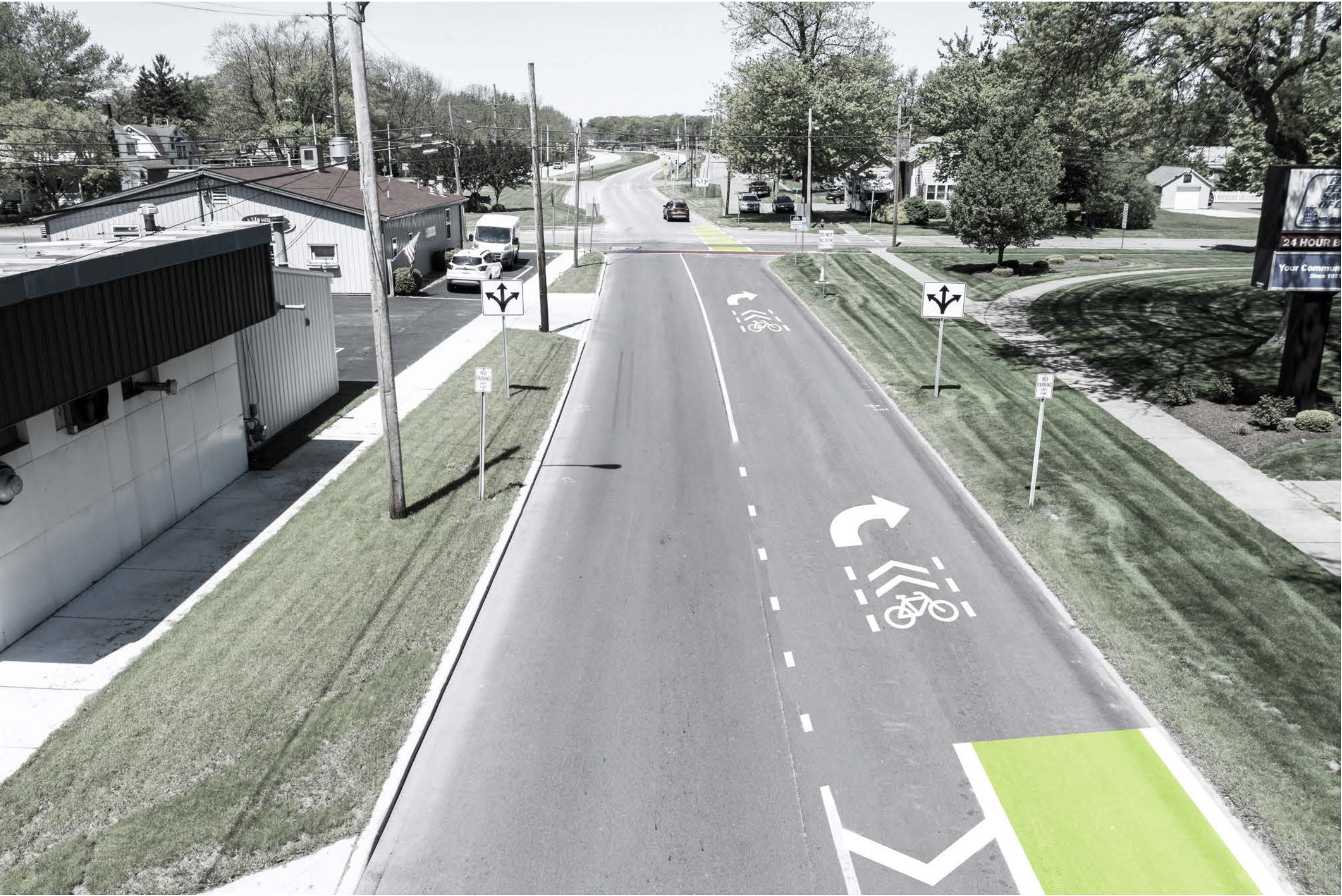
Painted bike lane delineation looking west toward Williams St. The bike lane ends as indicated by striping through the Williams St intersection. Note the updated shared turn lane onto Williams.
