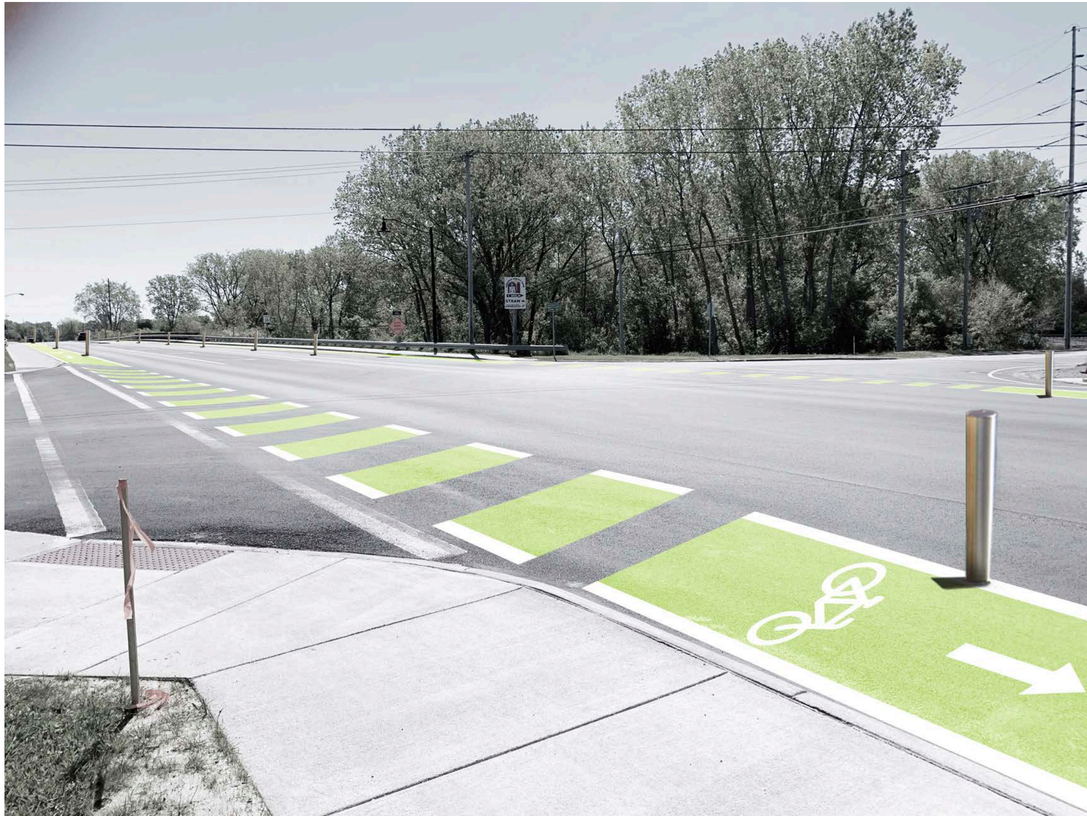
Painted striped bike lane adjacent to crosswalk at the intersection of River Rd and US 6 looking southeast toward Berlin Rd
