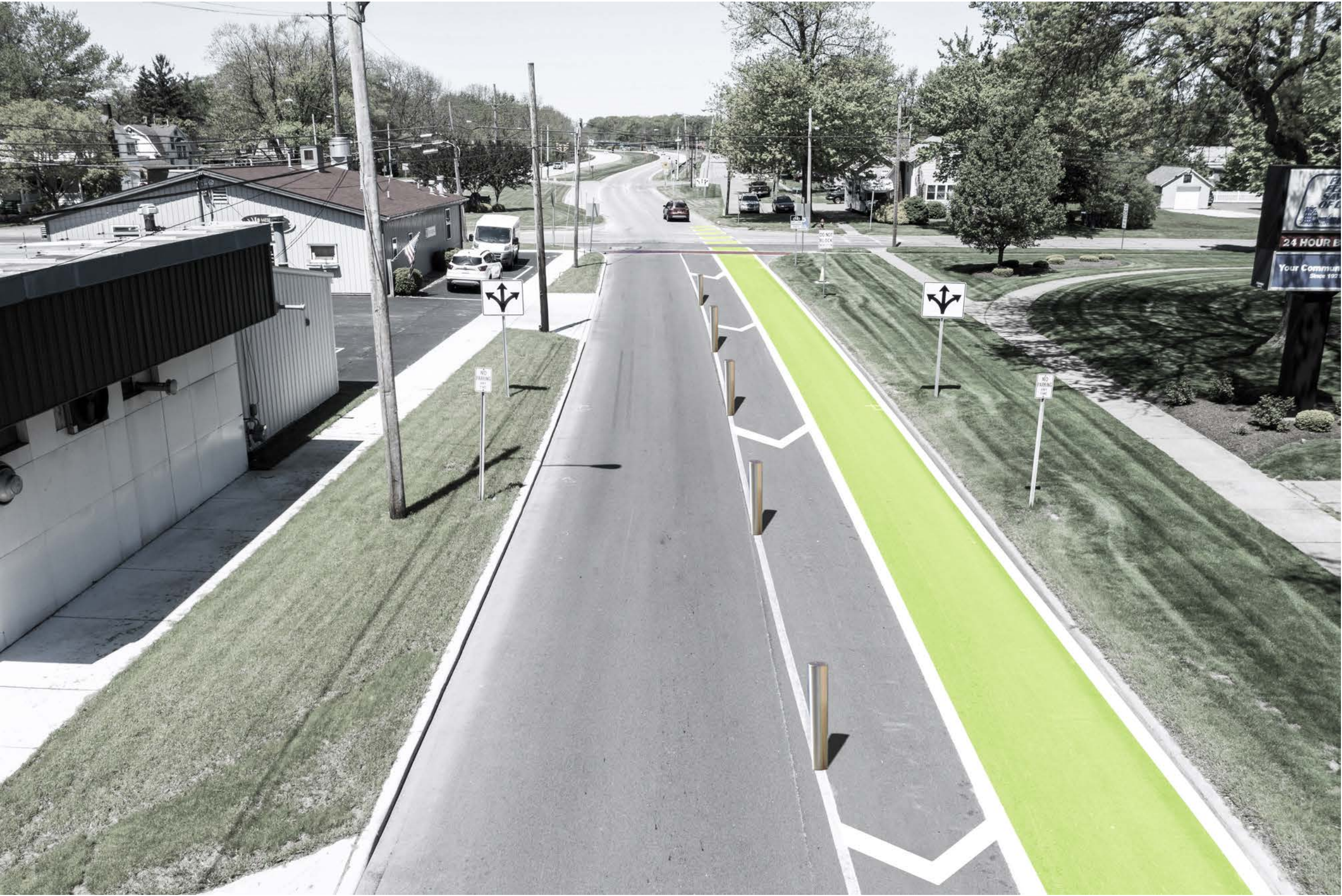
Painted bike lane delineation with bollards looking west toward Williams St. The bike lane ends as indicated by striping through the Williams St intersection
