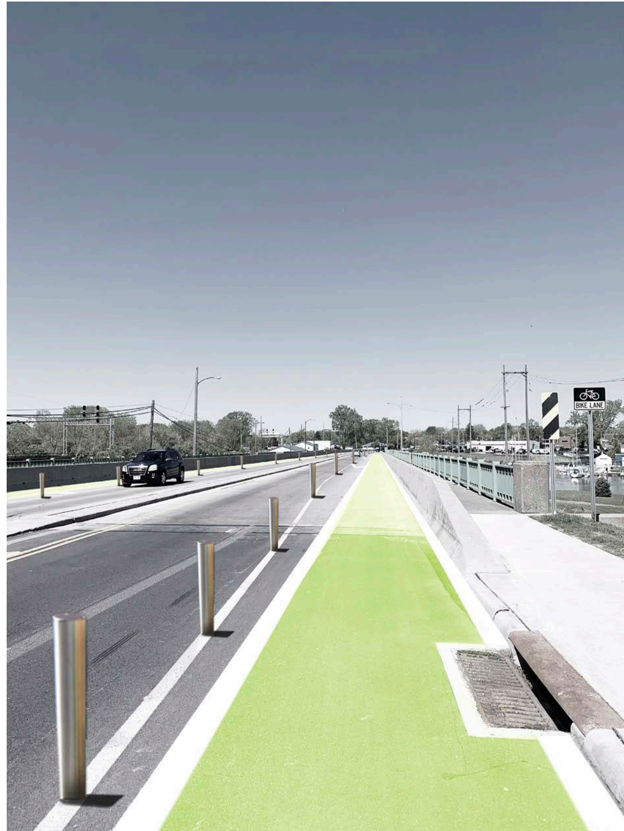
Painted bike lane delineation with buffer/bollards approaching the Huron River bridge - view looking west toward Downtown
