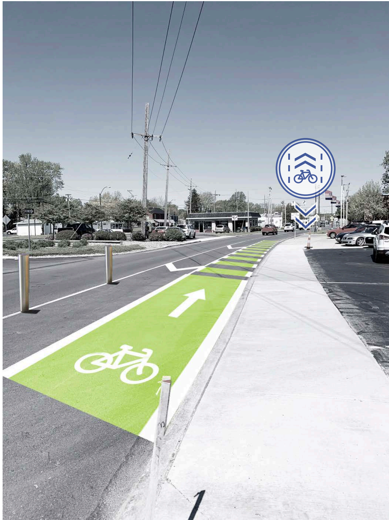
Painted bike lane delineation with bollards looking west toward Huron Street. The lane is condensed into a sharrow within the right turn lane.
