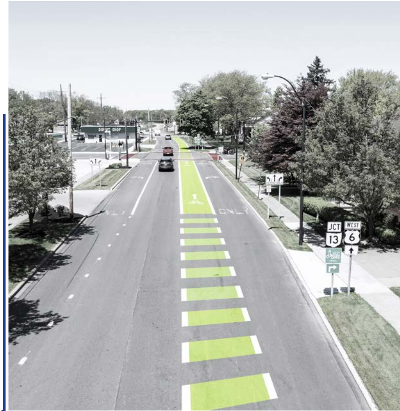
US 6 looking west toward Main St
