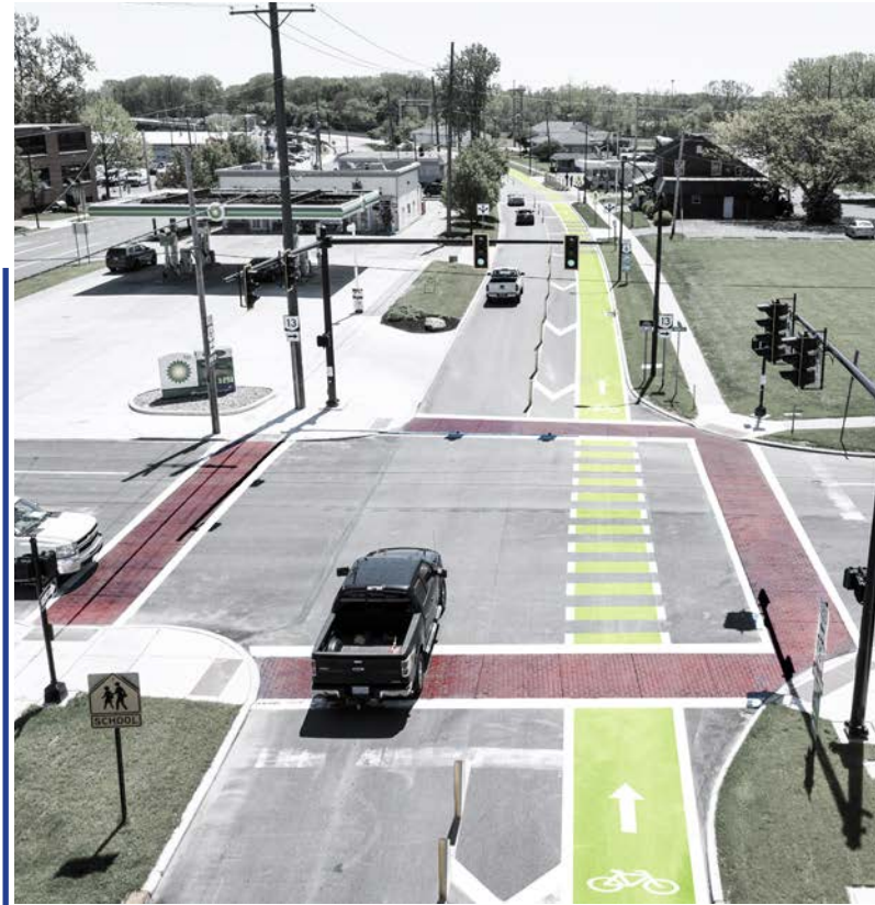
US 6 and Main St looking east toward Huron River bridge
