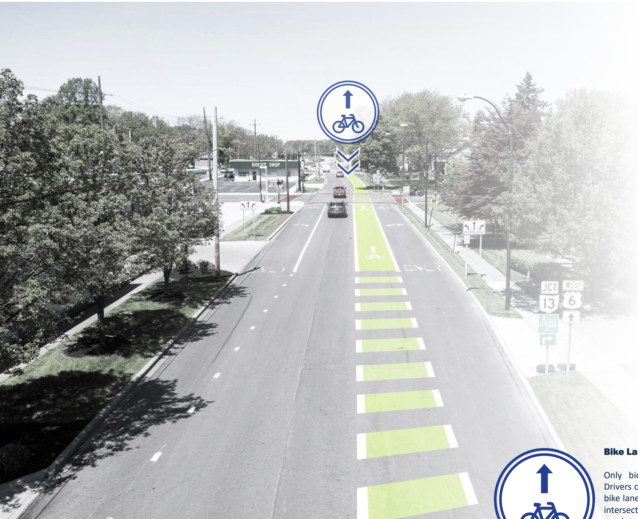
Painted striped lane delineation looking west toward Main St. Dashed lines indicate vehicular merging
