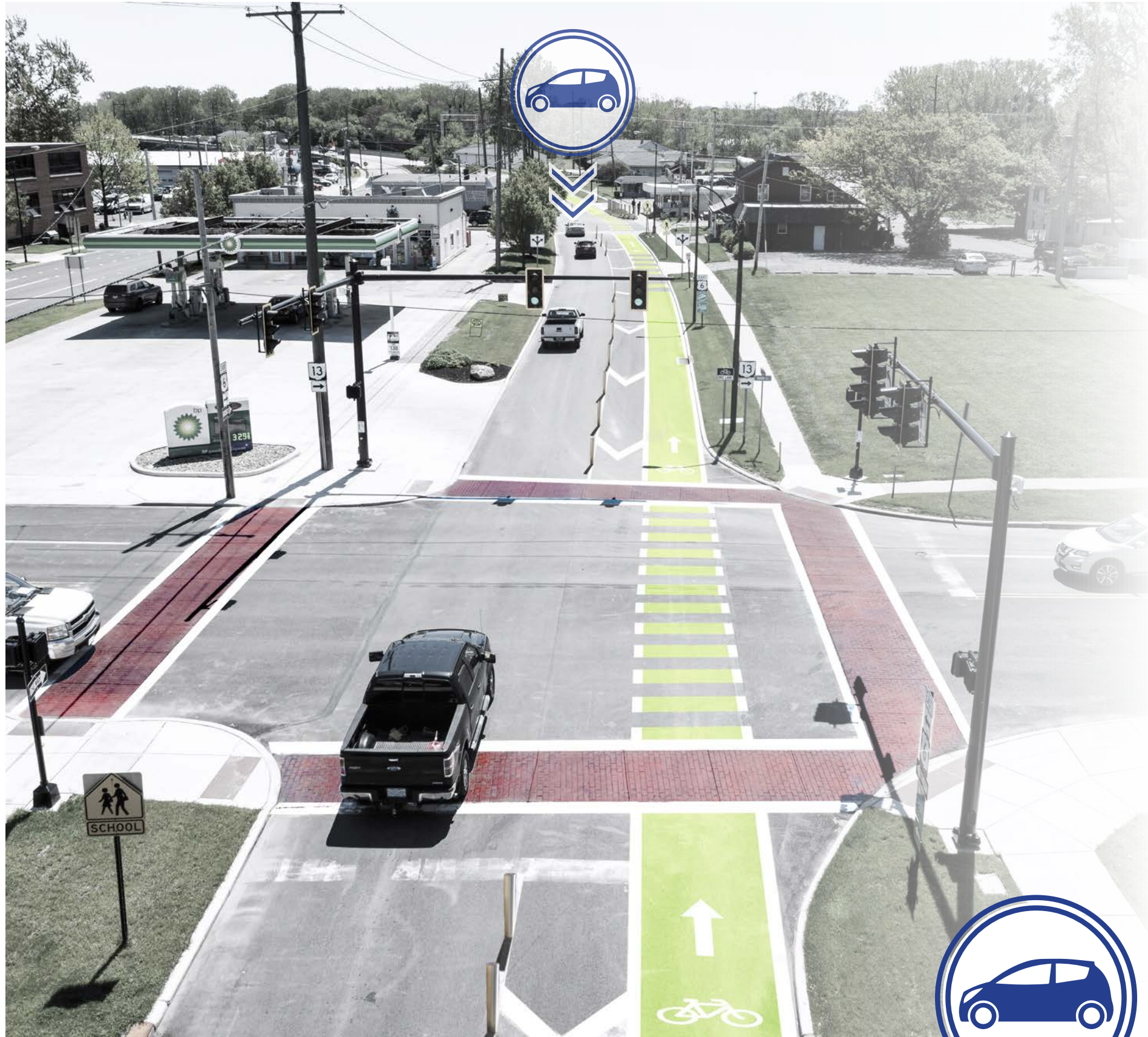
Painted bike lane delineation with bollards at Main St looking east. The view shows the bike striping through intersections in relation to crosswalks.
