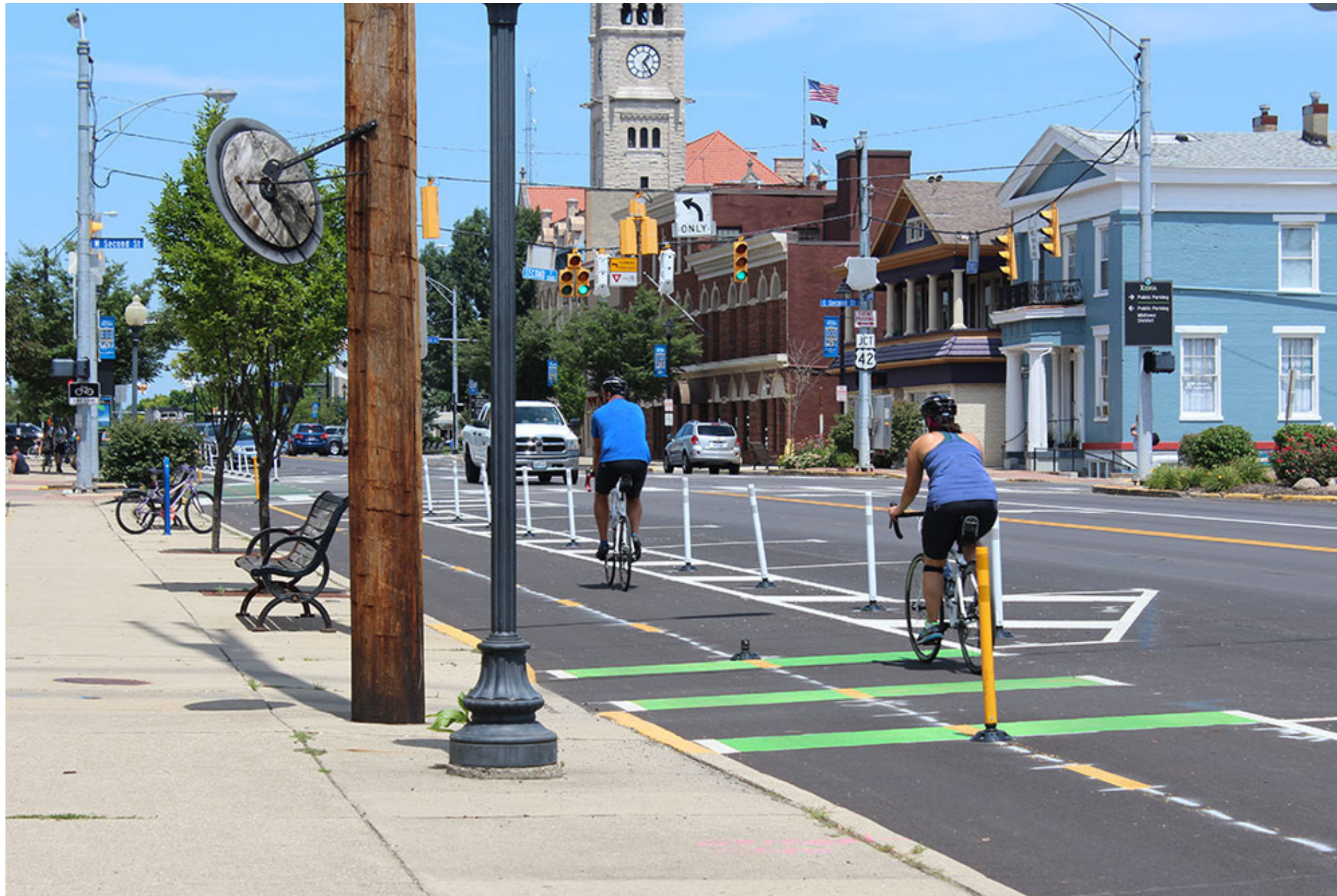
Protected cycle track through downtown Xenia, OH featuring enhanced striping and bollards to further emphasize safety and delineate bike lane space
