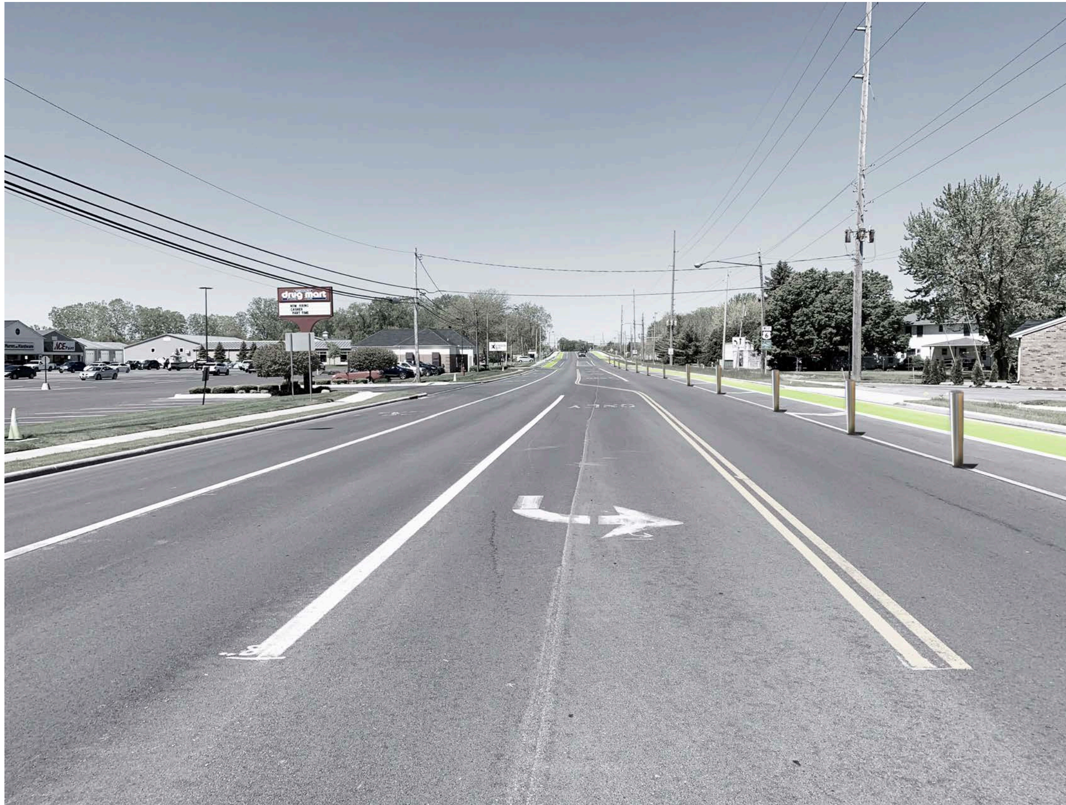
Painted striping and bollards to indicate delineation of separate protected bike lane from motorist traffic at the intersection of Berlin Rd - view looking west toward Downtown
