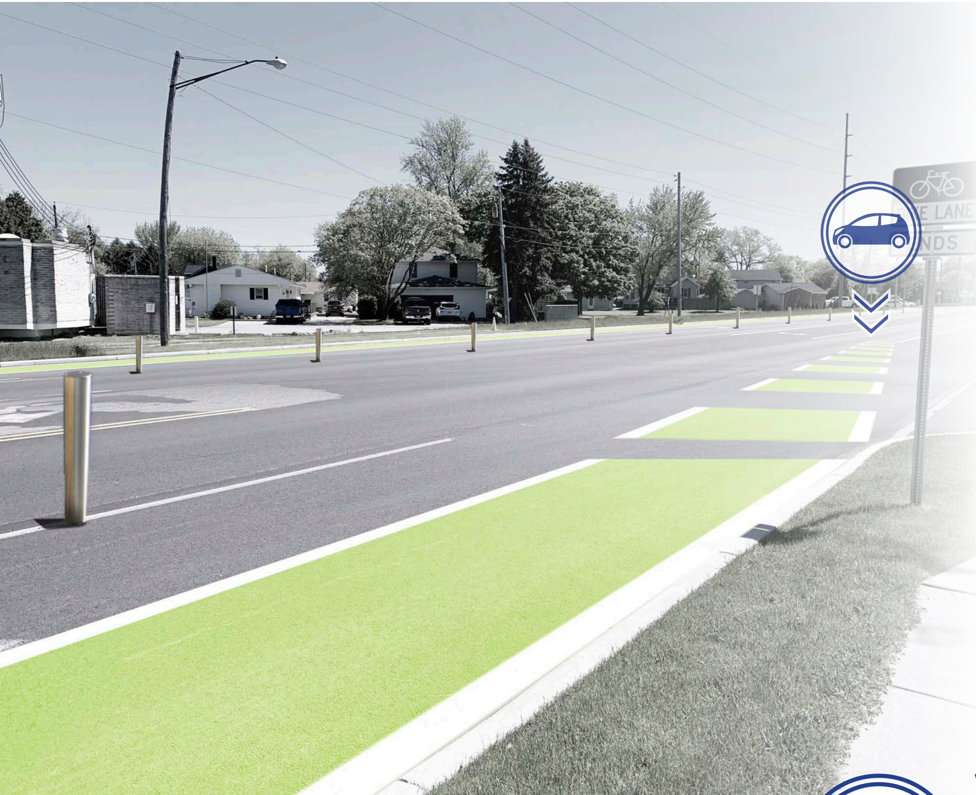
Painted striping to indicate merging of the bike lane back into motorist traffic - looking east at the Commerce Plaza entrance - view looking toward Berlin Rd
