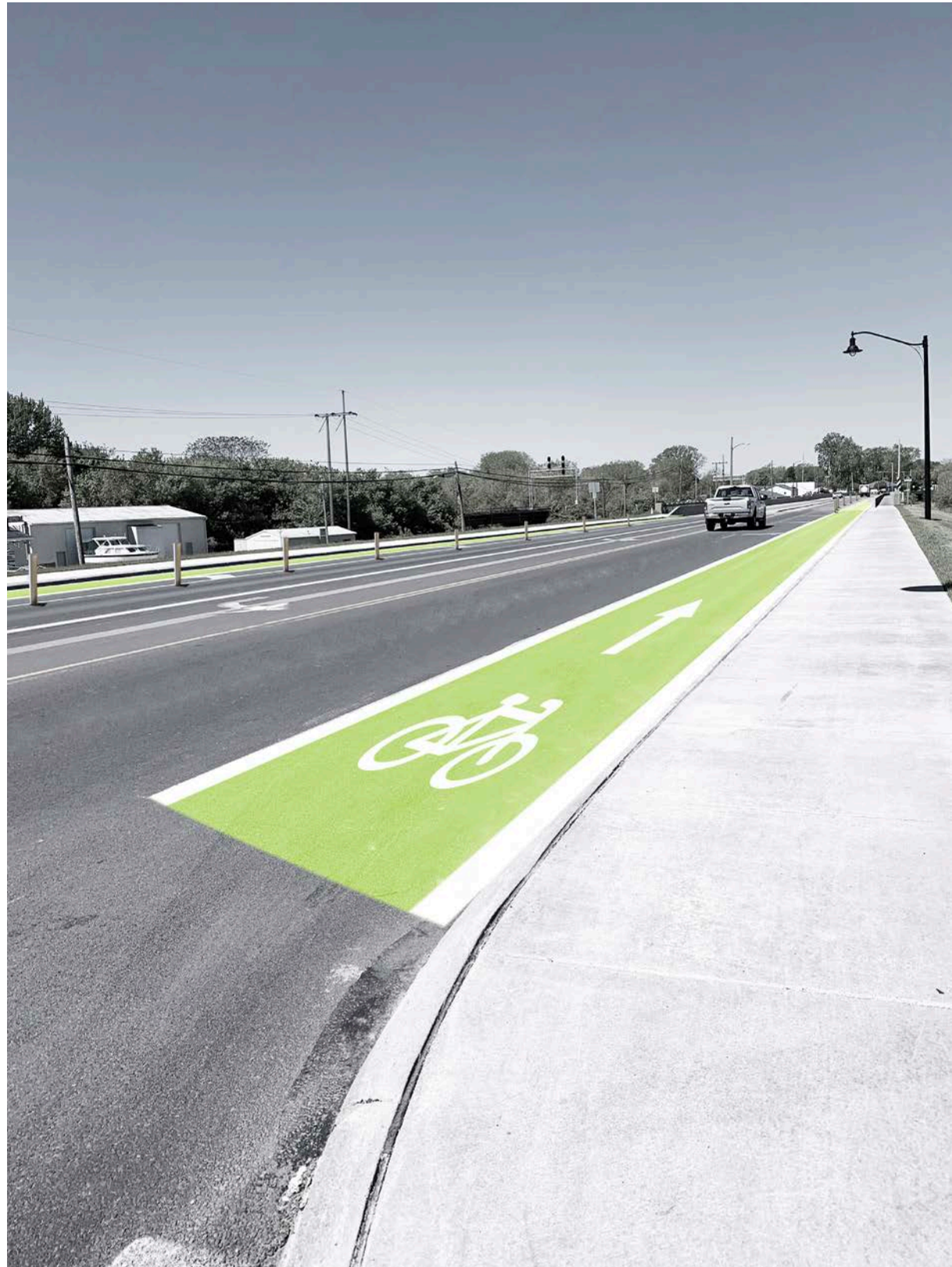
Painted bike lane delineation at the intersection of River Rd and US 6 looking west toward Downtown
